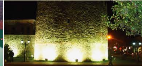
Works for the Lighting of the Walls of the Castles, under contract with Albanian Development Fond
